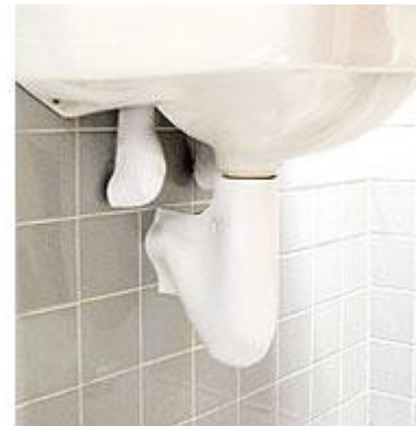
Diagram M – Pipe Insulation
