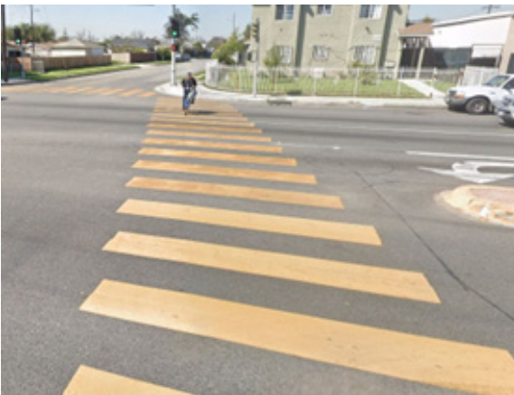
An example of a high-visibility continental crosswalk
