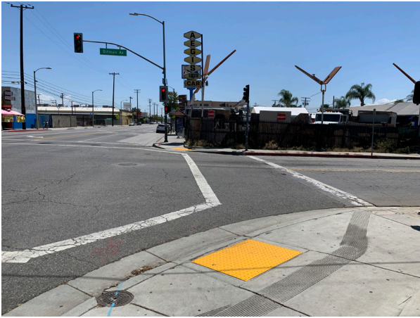
A standard crosswalk with two parallel lines and an ADA compliant curb ramp, East Los Angeles
