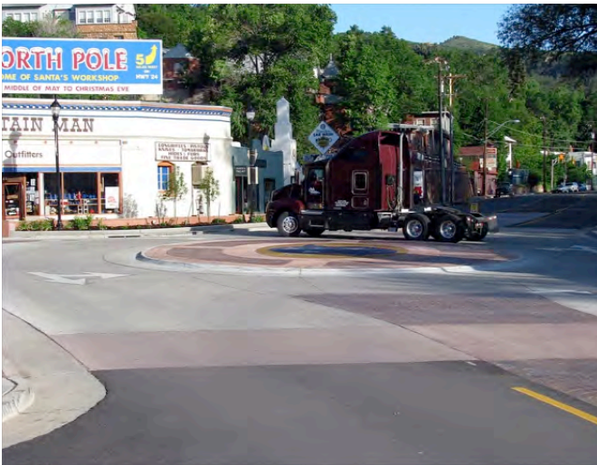
Mini-roundabout (Credit: Ian Lockwood)
