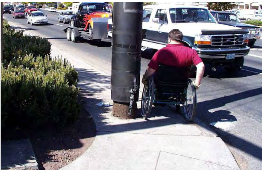
Obstructions can make passage difficult or impossible for wheelchair users (Credit: Michael Ronkin)
