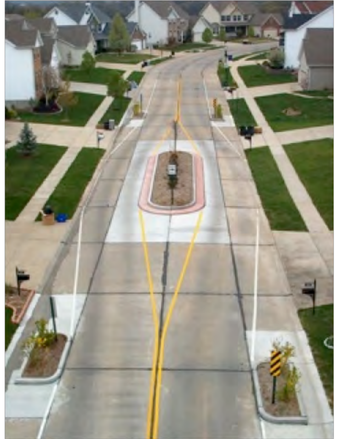
Oval median with tree wells. (Credit: Gary Crammer)
