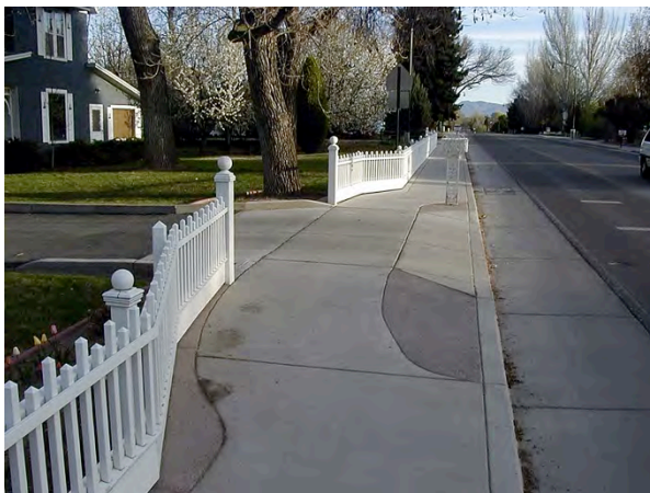
Routing sidewalks around driveway ramps maintains a flush surface (Credit: Dan Burden)
