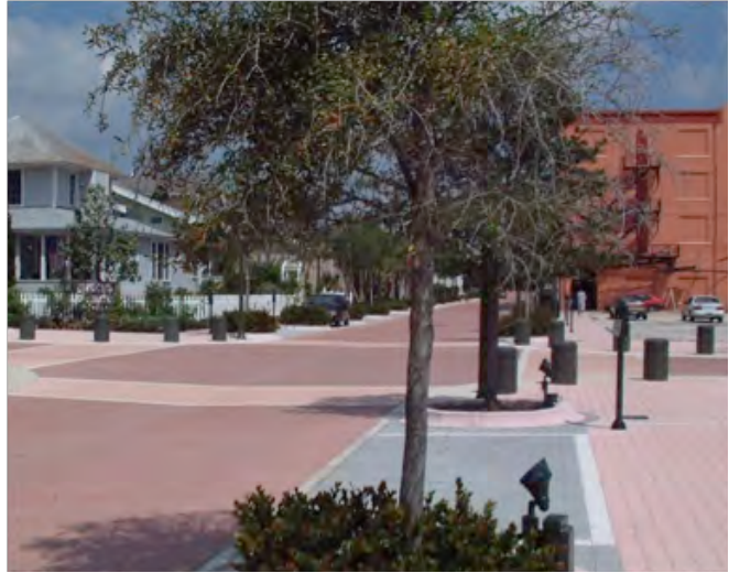
Textured pavement (Credit: Ian Lockwood)
