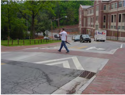
Raised crosswalk: University of North Carolina Campus, Chapel Hill, NC (Credit: Ryan Snyder)
