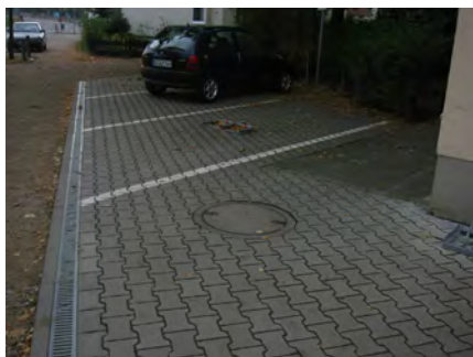
Permeable paving and a trench drain in a parking area (Credit: Stephanie Landregan)
