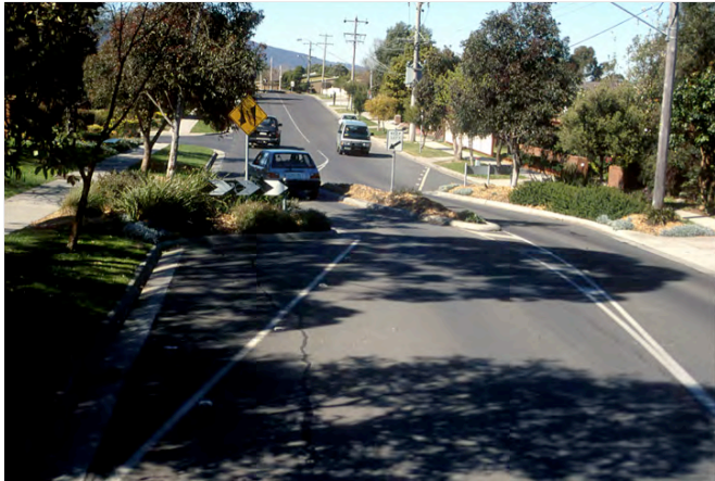
Two-lane chicane (Credit: Michael Wallwork)
