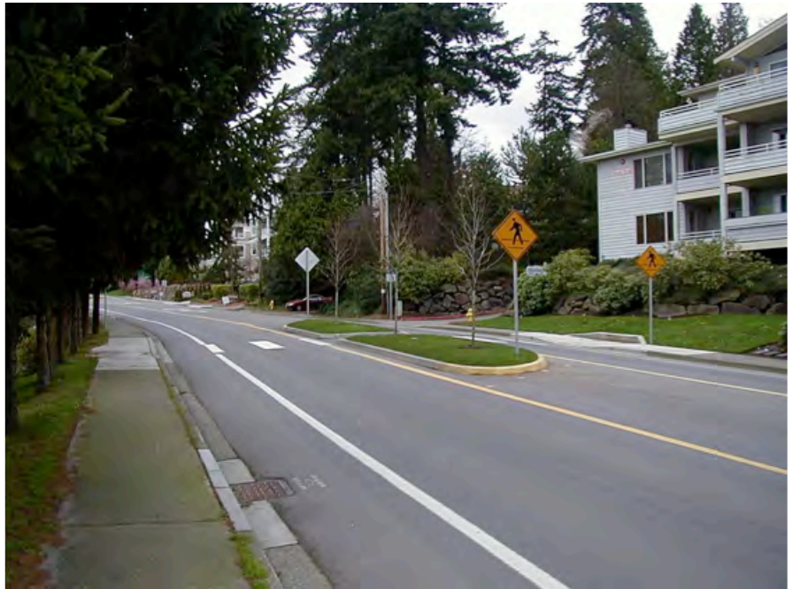
Midblock crosswalk (Credit: Dan Burden)
