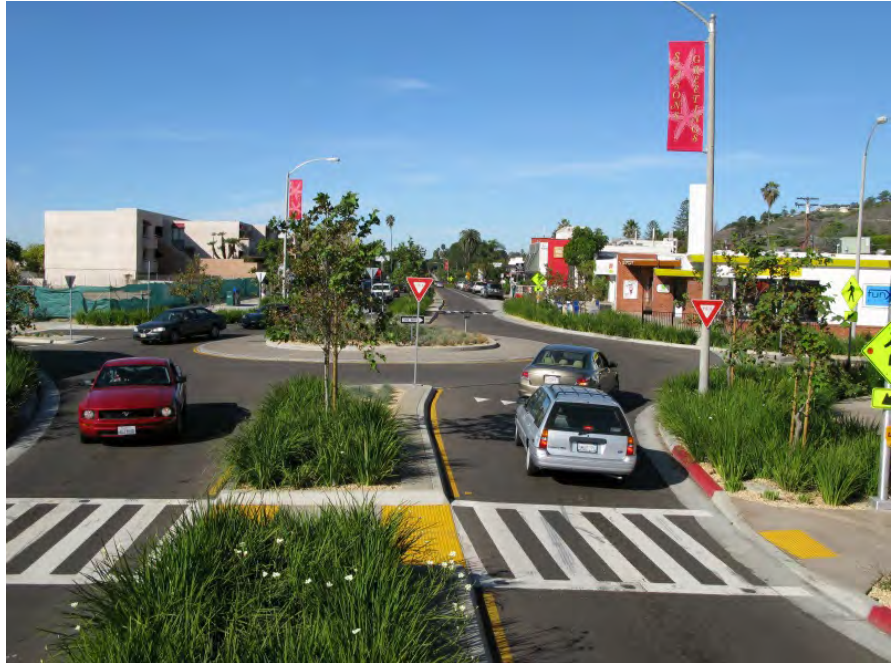
Roundabout: San Diego, CA (Credit: Michael Wallwork)
