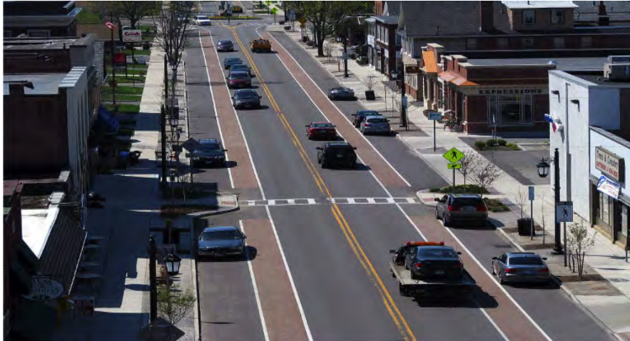
Parking assist lane (Credit: Michael Wallwork)
