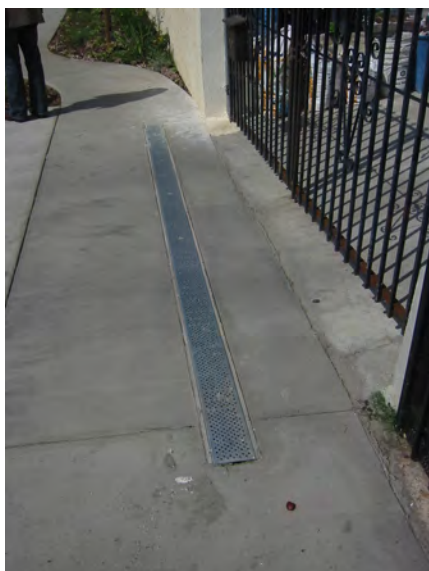
Trench drain in hardscape (Credit: Stephanie Landregan)
