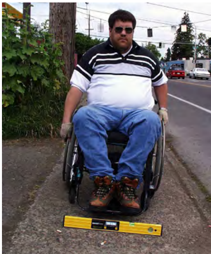
Steep cross slopes create difficulties for wheelchair users (Credit: Michael Ronkin)
