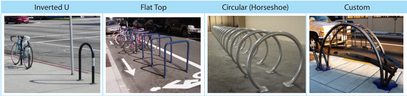
Figure G-1 Recommended Types of Short-Term Bicycle Parking
